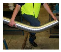
2/ Fit flue pipe to appliance (unsleeved end of flue). Insert flue connection fully into flue pipe. Fit hose clamp to connection and tighten.
