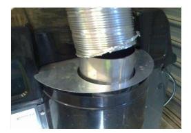
3/ Form extra bends where required. Care should be taken when forming bends to not create a low point where condensation may collect. Condensation should be able to drain to the heater or out the flue outlet.
