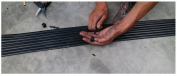
**STEP 5:** Place a pressure sleeve on either side of the collector.
