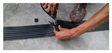
**STEP 2:** Cut the webbing between the tubes on either side of the hole.
