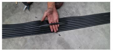
**STEP 7:** Push the other side of the collector over the joining barb to connect the two sides.
